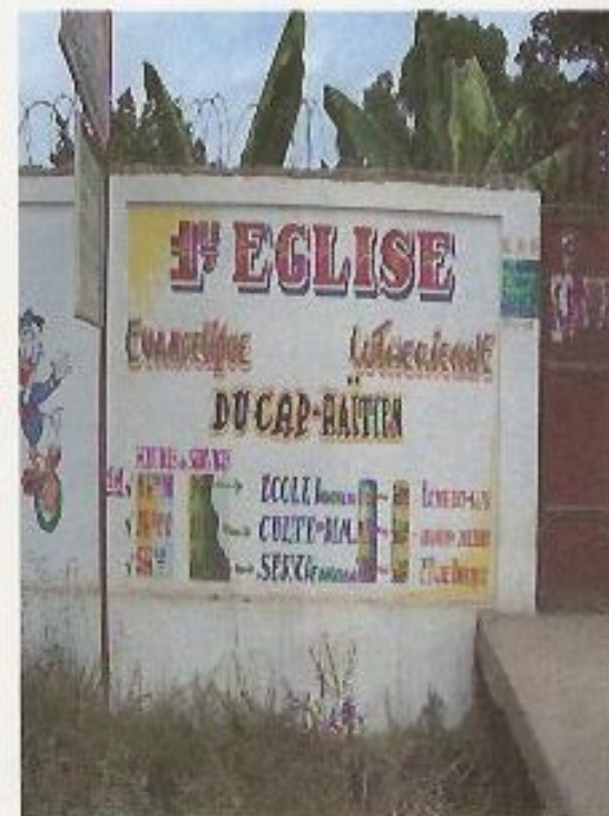
The entrance to First Lutheran Church of Cap Haitian.
